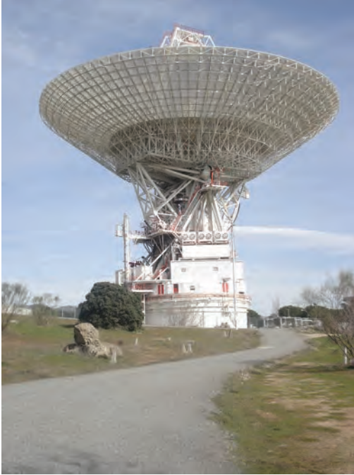
Deep Space Station-63 (DSS-63) at Madrid Deep Space Network Complex.
