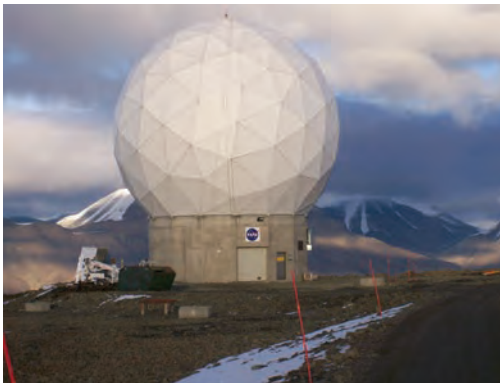
A close-up of one of the six radomes at SvalSat.
